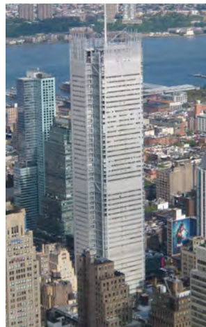
NY TIMES building レンゾピアノ
